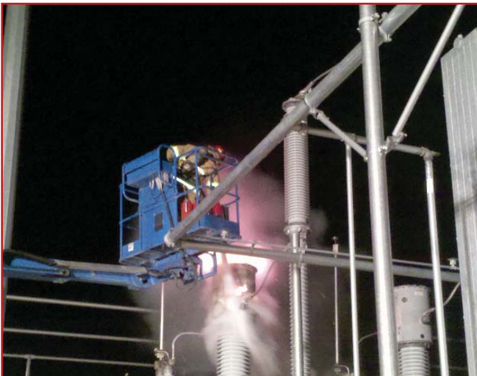
Applying Three ABC Extinguishers
