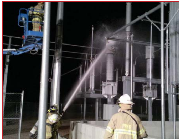
F-500 EA - Extinguished in 20 Seconds
